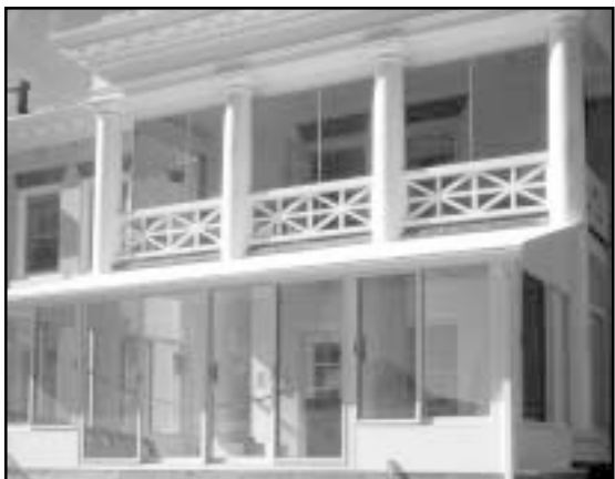
The new sun porch at the Deaconess is well under way.
